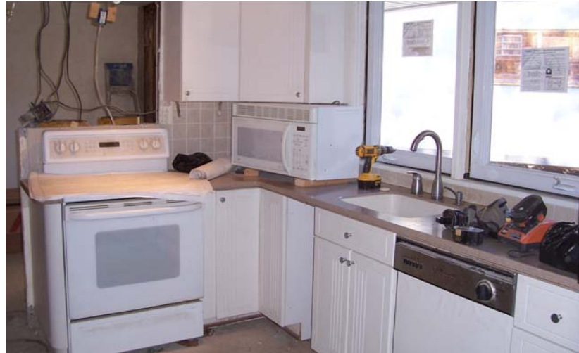
Renovation of the kitchen in progress
