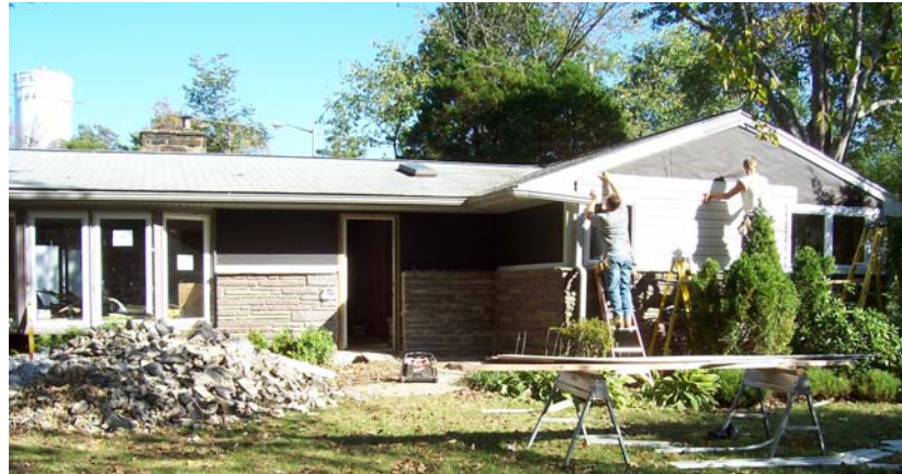
Construction of HomeWorks, before staging area was installed
