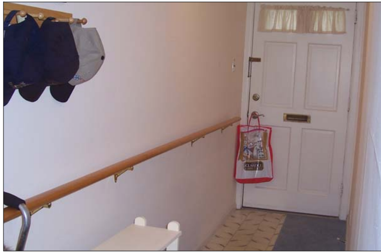
An inside railing was installed down the length of the hallway.
