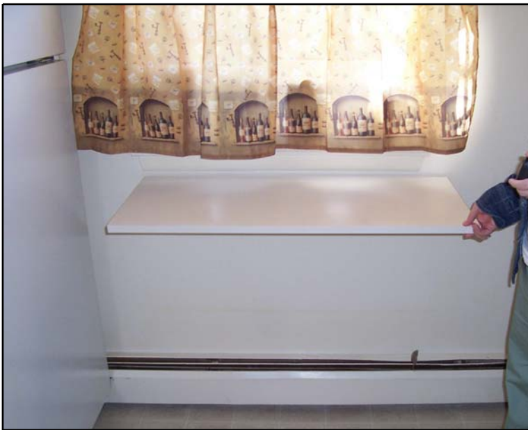
A pull-down table was installed in Mr. Warren's kitchen to allow for a wheelchair and preserve space
